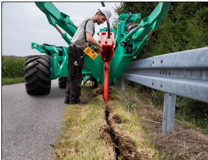
pic 1. The FOECK laying plough FSP 6 allows the installation directly at the property boundary. It is operated with the radio remote control FRC 2-1.
