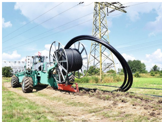
Trenchless laying of power lines with the world's most efficient laying system from FOECK
